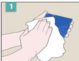
Wipe and thoroughly clean back of each tile prior to application of setting material. Please see important note above.
